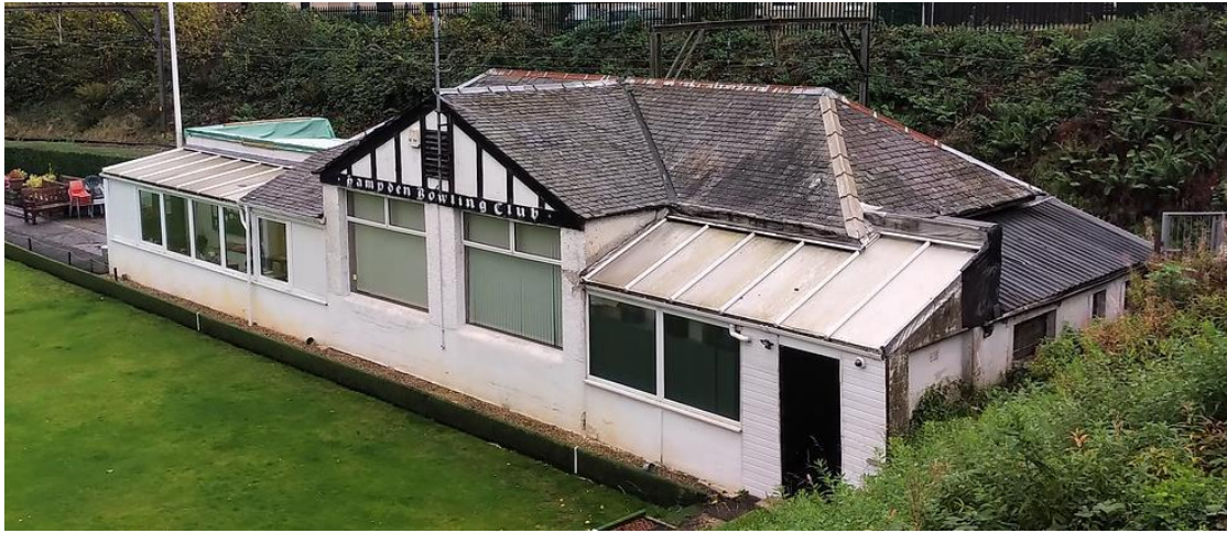
Contemporary view of the Hampden Bowling Club pavilion, front.
